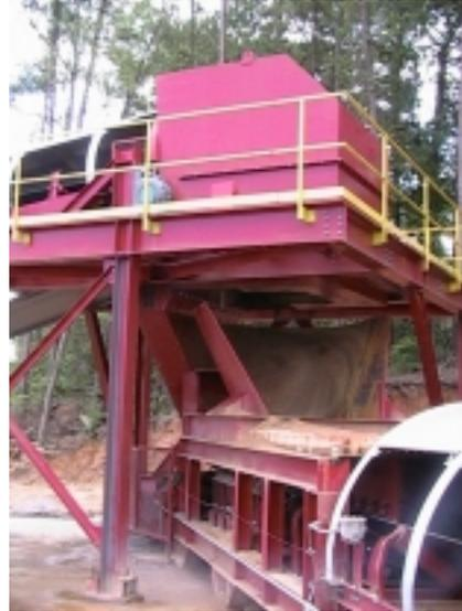
Figure 21 - Conveyor 5 to 6, 72-inch wide belt conveyor system, transfer point as it was being installed.
