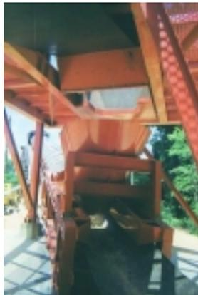
Figure 20 - Conveyor 6 to 7, 72-inch wide belt conveyor system, transfer point as it was being installed.
